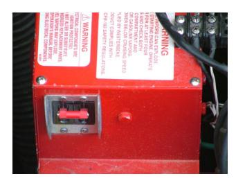
When generator is running and the Inverter is on, should be 12.5 volts or greater and you should show 120 volts on the meters on the breaker panel.
